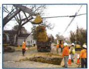
Removal of Manhole to be Replaced Williamston, NC
