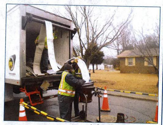
Installation of CIPP Sewer Liner, Williamston, NC
