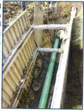
Installation of Point Repair Prior to Pipeline Lining Vanceboro, NC
