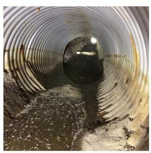
20 linear feet of 60" CMP replacement due to failure exceeds \$20,000.
